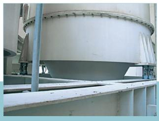
The precise compression load cells PR 6201 are specially designed for the weighing of silos, tanks and vessels
