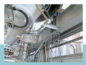
The transmitter was connected to the load cells through a 6-wire connection
